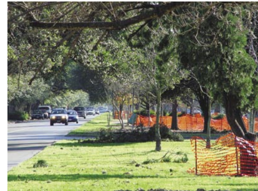
Houston Heights esplanade jogging trail is being renovated.
