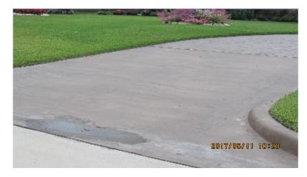
**Option 2**: Grade the subgrade to proper slope and form the driveway to meet the new grades /slope. You would see the finished dirt with the proper slope. Homeowner will finish the driveway with their desired finish at their cost. (Driveway must be finished 2 weeks after it's been prepped by the City.)
