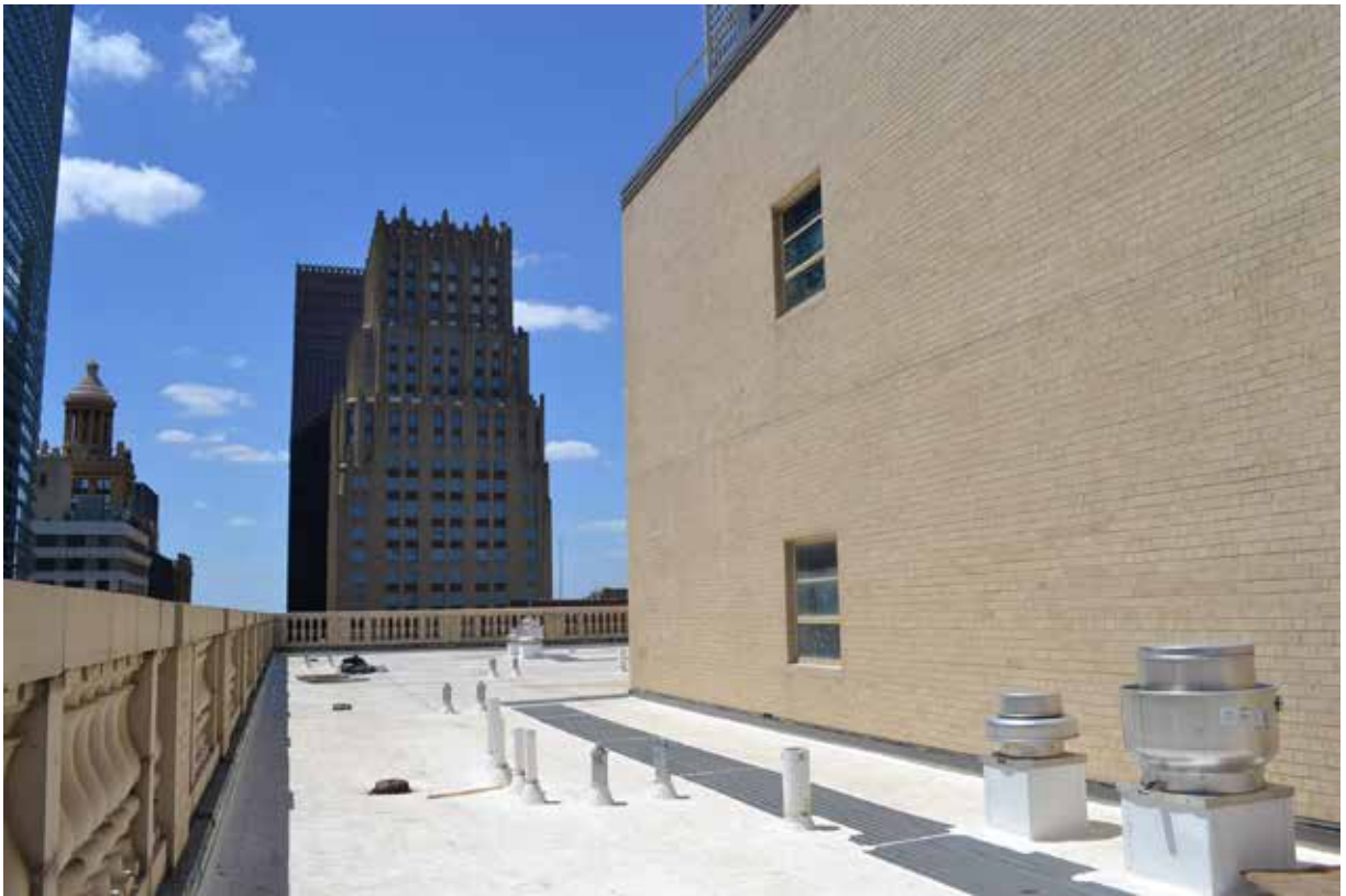
A: Roof, S elevation of 1959 penthouse, view W June, 2017
