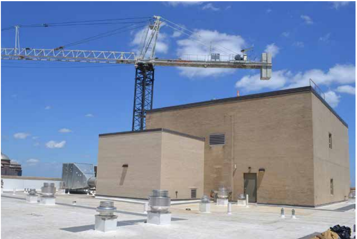
A: Roof, overall of 1959 roof penthouse (in rear) and new mechanical addition, view NE June, 2017
