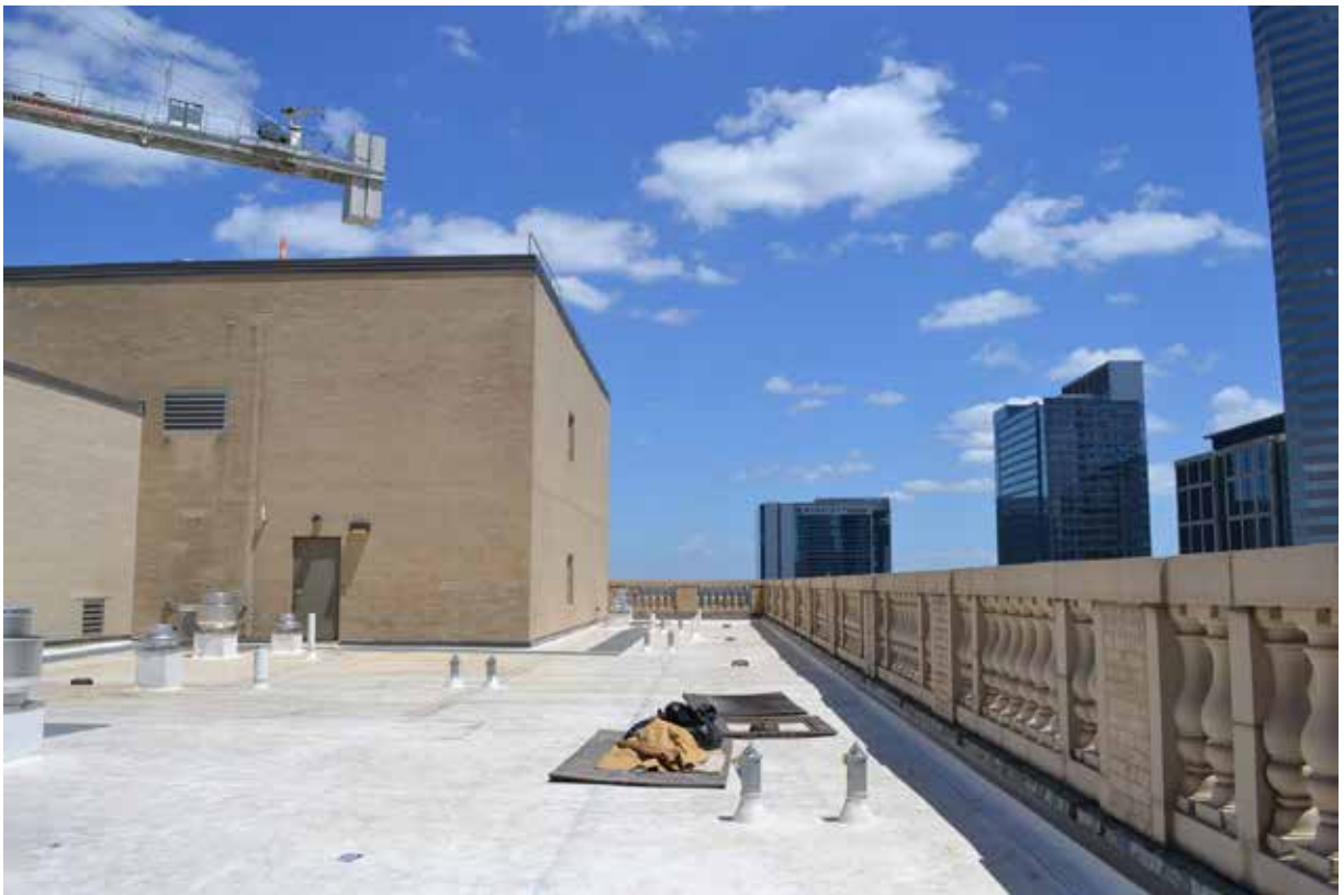
B: Roof, S elevation of 1959 penthouse, view E June, 2017
