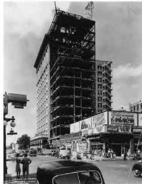
VIEW SOUTH DOWN SAN JACINTO STREET OF CONSTRUCTION OF 1936 BUILDING ADDITION (COURTESY OF AVERY ARCHITECTURAL AND FINE ARTS LIBRARY, COLUMBIA UNIVERSITY, NY, NY)
