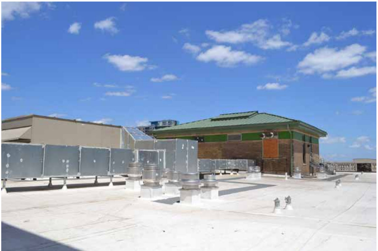
B: Roof, overall, view NE, new duct work and 1915 penthouse June, 2017
