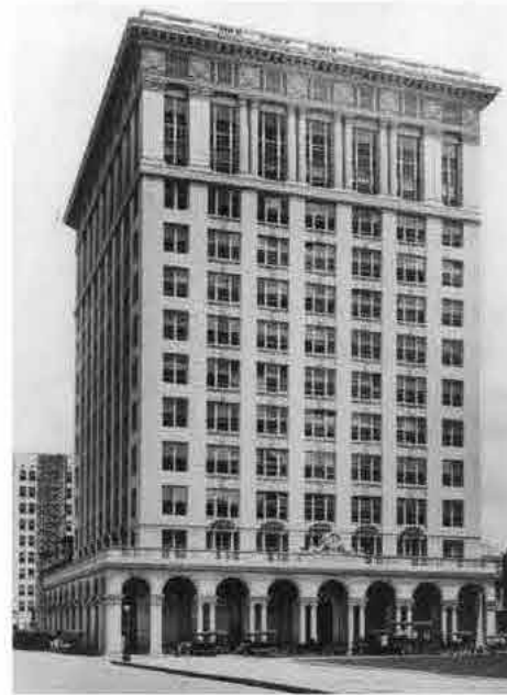
EAST AND SOUTH FACADES OF ORIGINAL 1915 BUILDING (COURTESY OF METROPOLITAN RESEARCH CENTER, HOUSTON PUBLIC LIBRARY)
