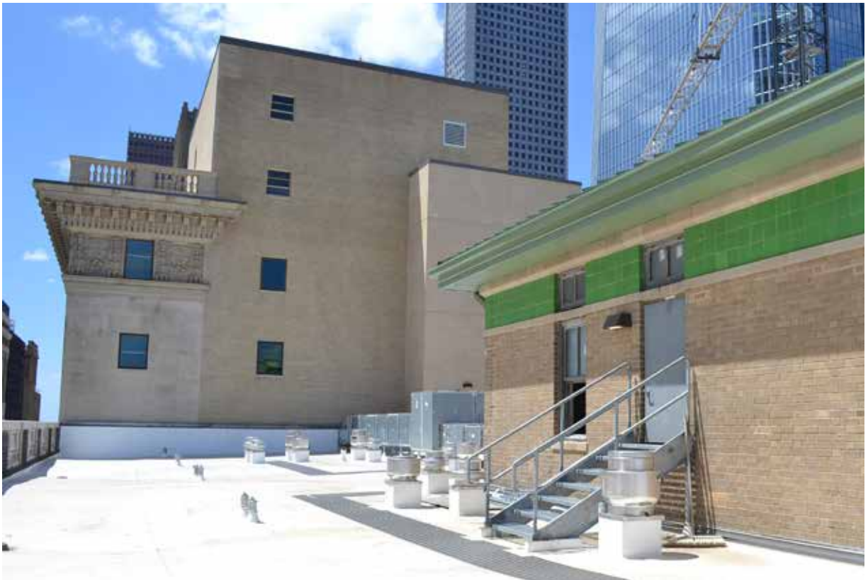
A: Roof, overall, view W from 1915 roof towards 1959 June, 2017
