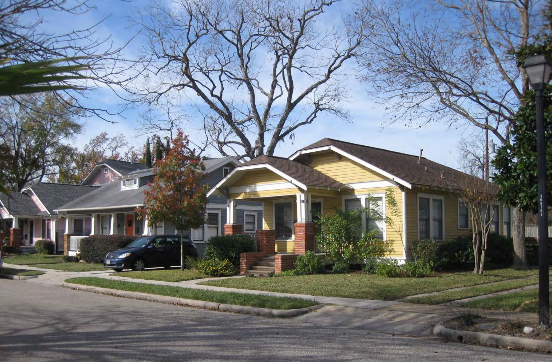
Residence, 1027 Key Street SE corner, looking NW
