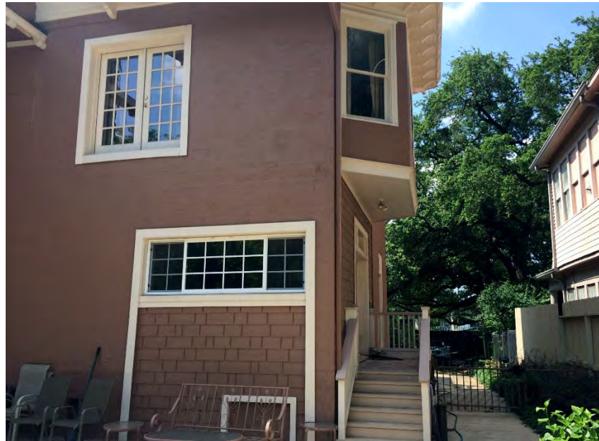
Original wood doors and transom within cementitious shake shingle infill
