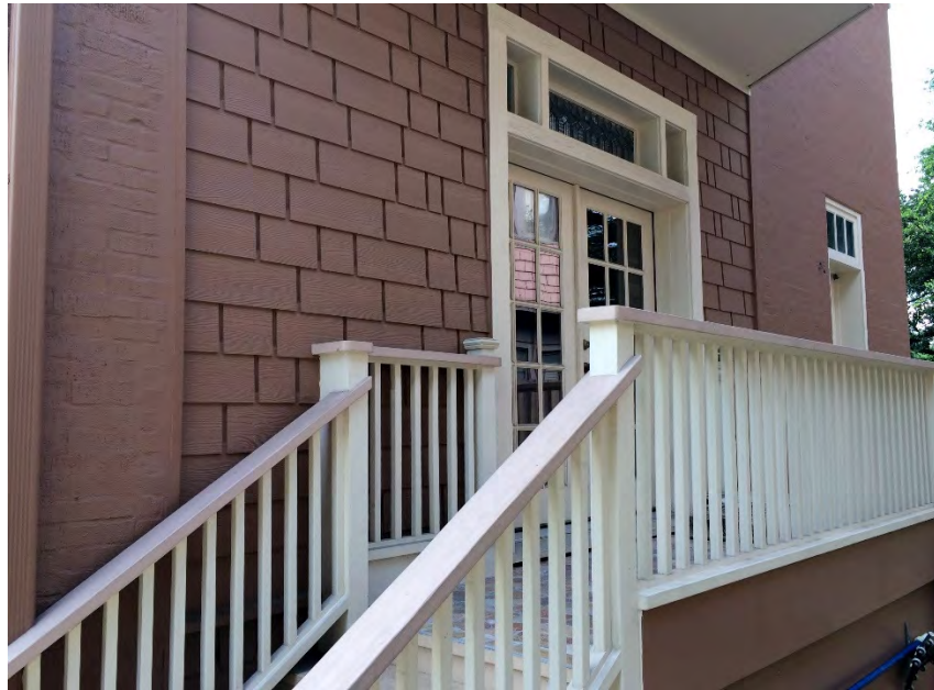
Original wood doors and transom within cementitious shake shingle infill
