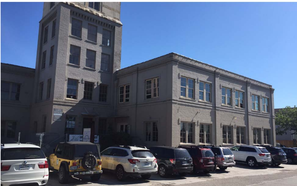
VIEW TOWARDS KRAFTSMEN BAKING ENTRANCE FROM W. 22 ND ST.
