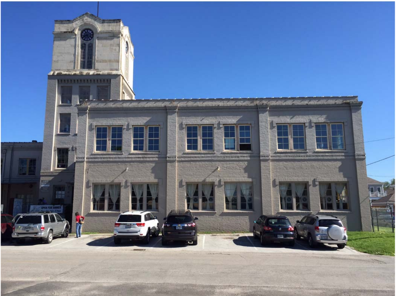
VIEW OF BUILDING ELEVATION FROM W. 22 ND ST.
