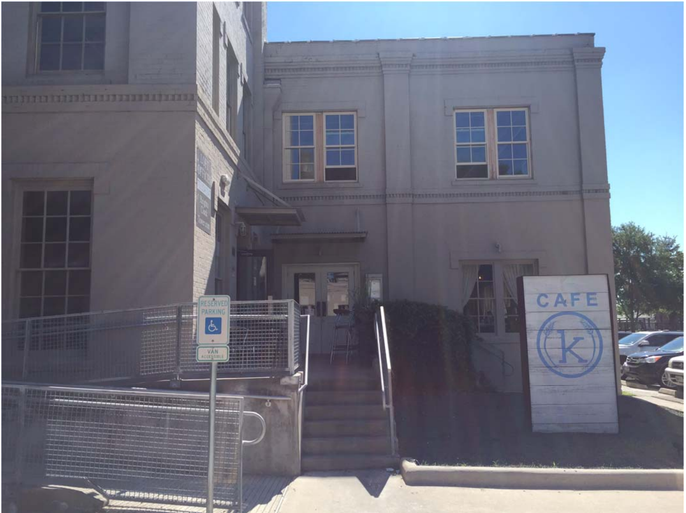
VIEW OF WESTERN BUILDING ELEVATION FROM SITE PARKING
