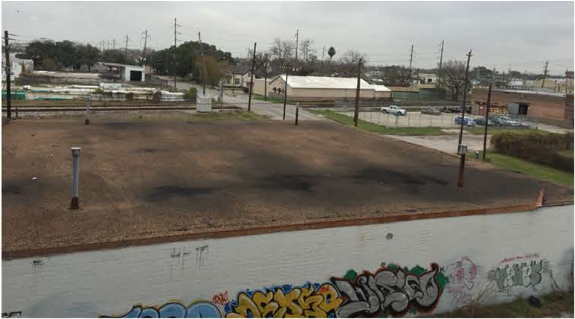
"BUILDING C" SOUTH FACADE
