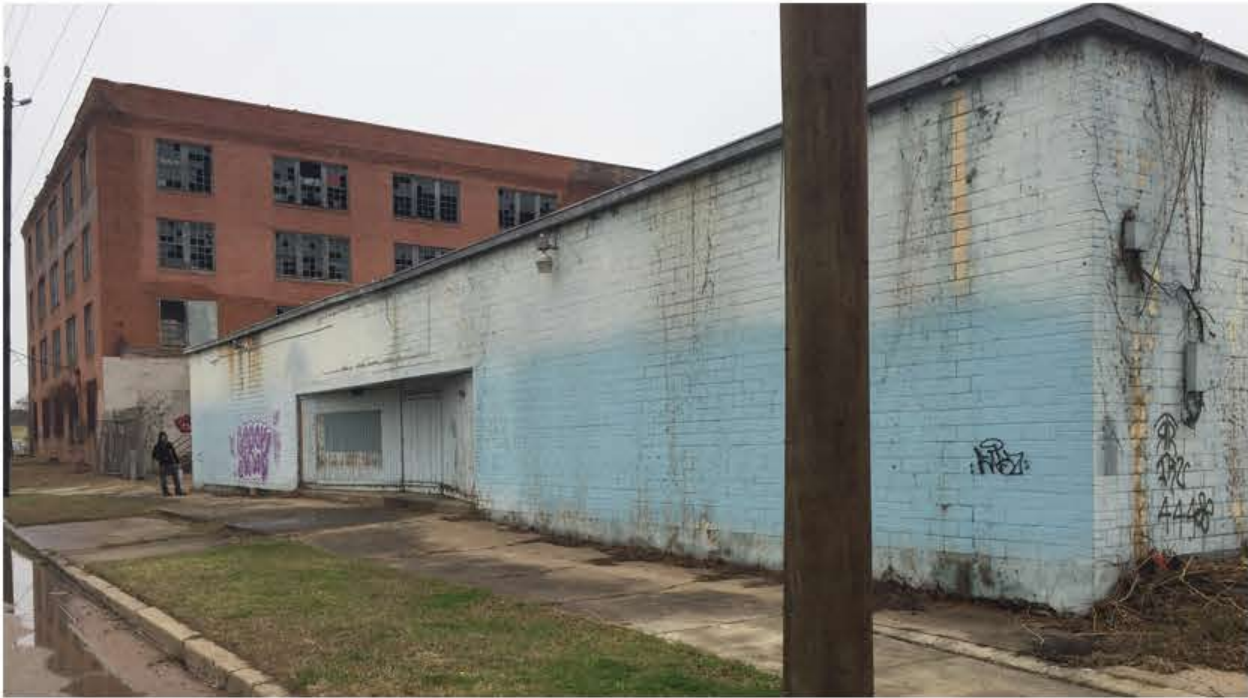
"BUILDING C" EAST FACADE
