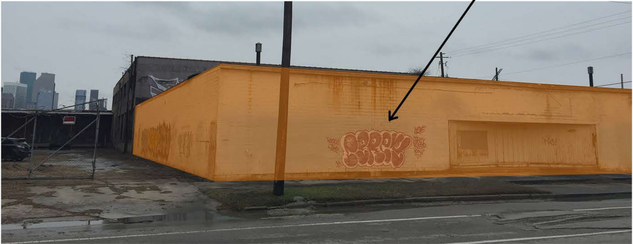
"BUILDING C" EAST FACADE
