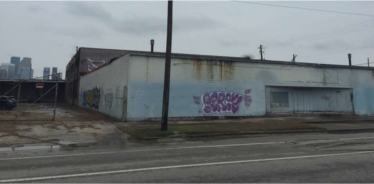
"BUILDING C" EAST FACADE
