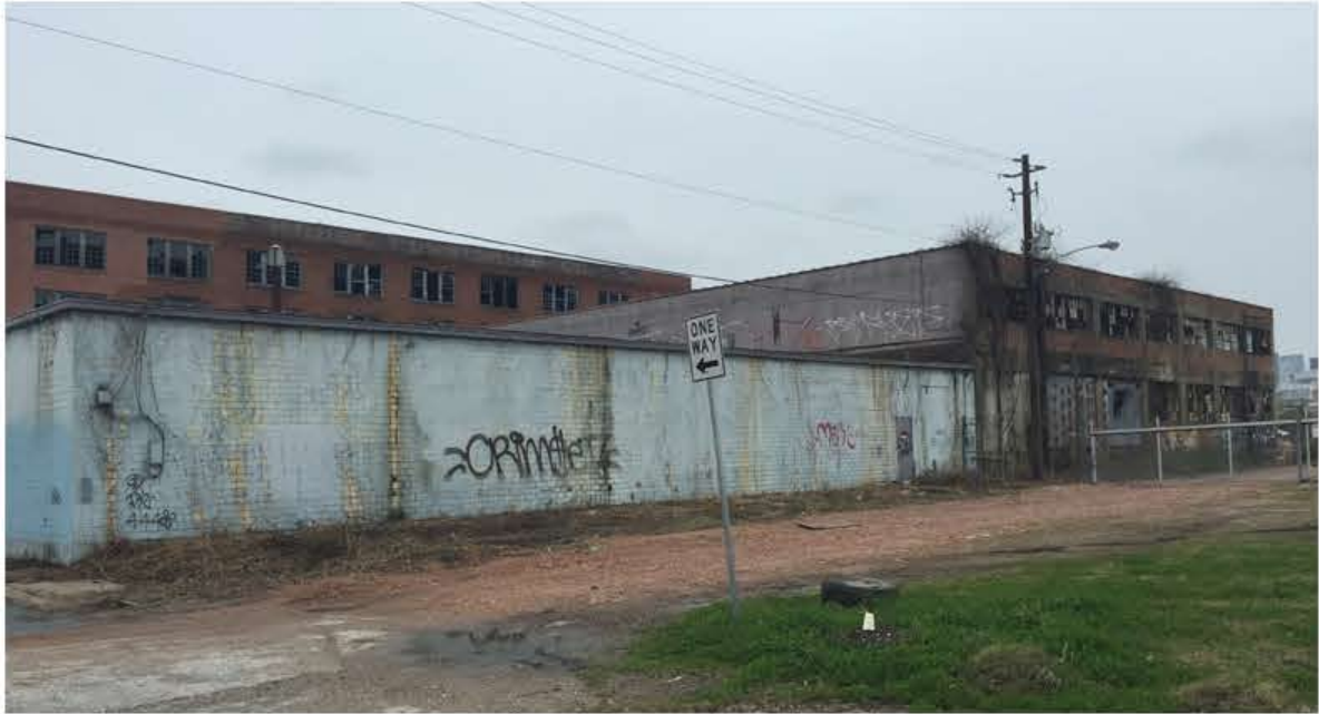
"BUILDING C" NORTH FACADE
