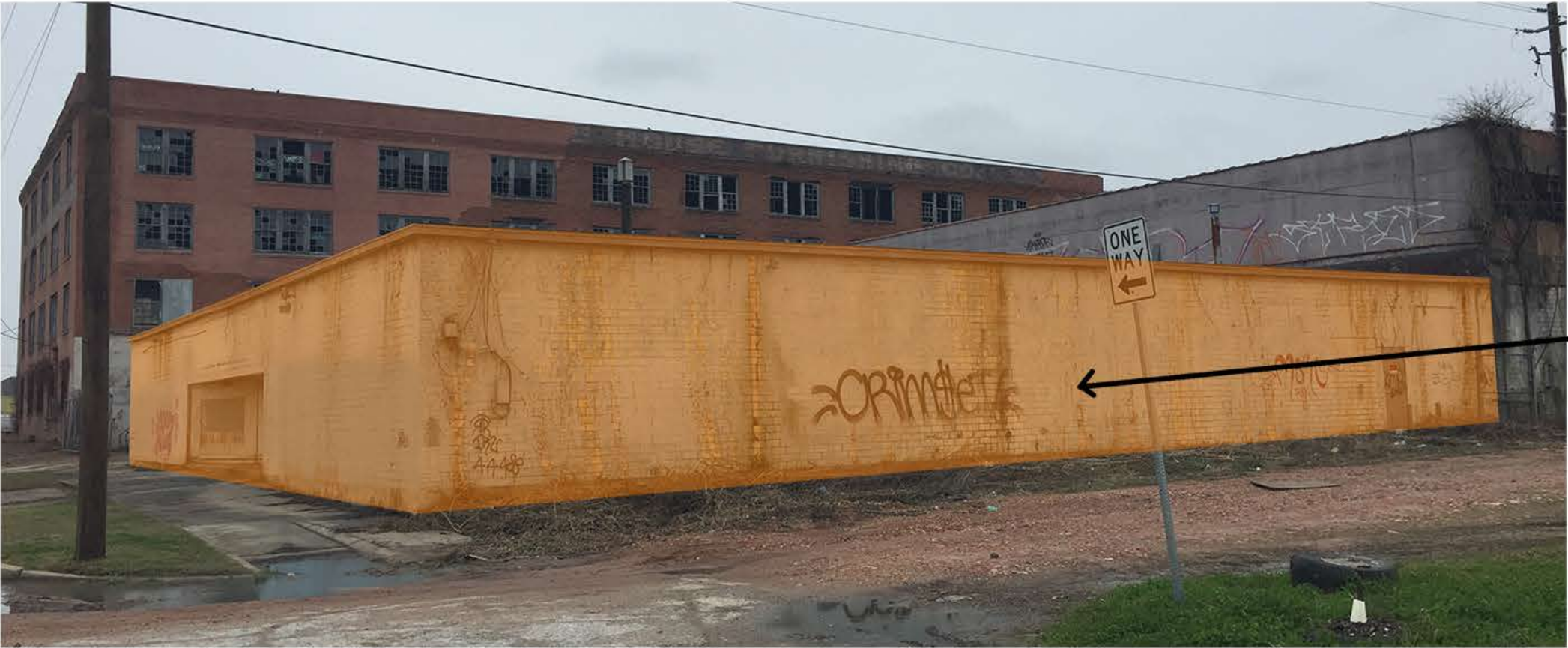
"BUILDING C" NORTH FACADE
