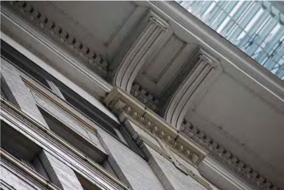
B: Detail of cornice and pilaster capitals. SWCA photo, 2014. _File: 00_DSC_0158
