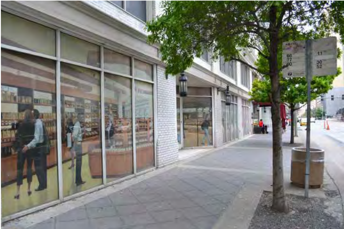
A: Detail east facade storefront, view N up Fannin. SWCA photo, 2015. File: 00_DSC_0001
