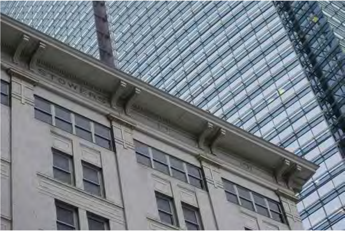
A: Detail of cornice, view NW. SWCA photo, 2014. File: 00_DSC_0157
