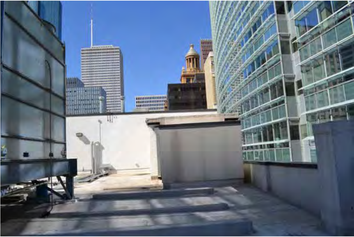
A: Roof, view W. East elevation of electrical closet in middle ground; mechanical penthouse in background. SWCA photo, 2014. File: 0672
