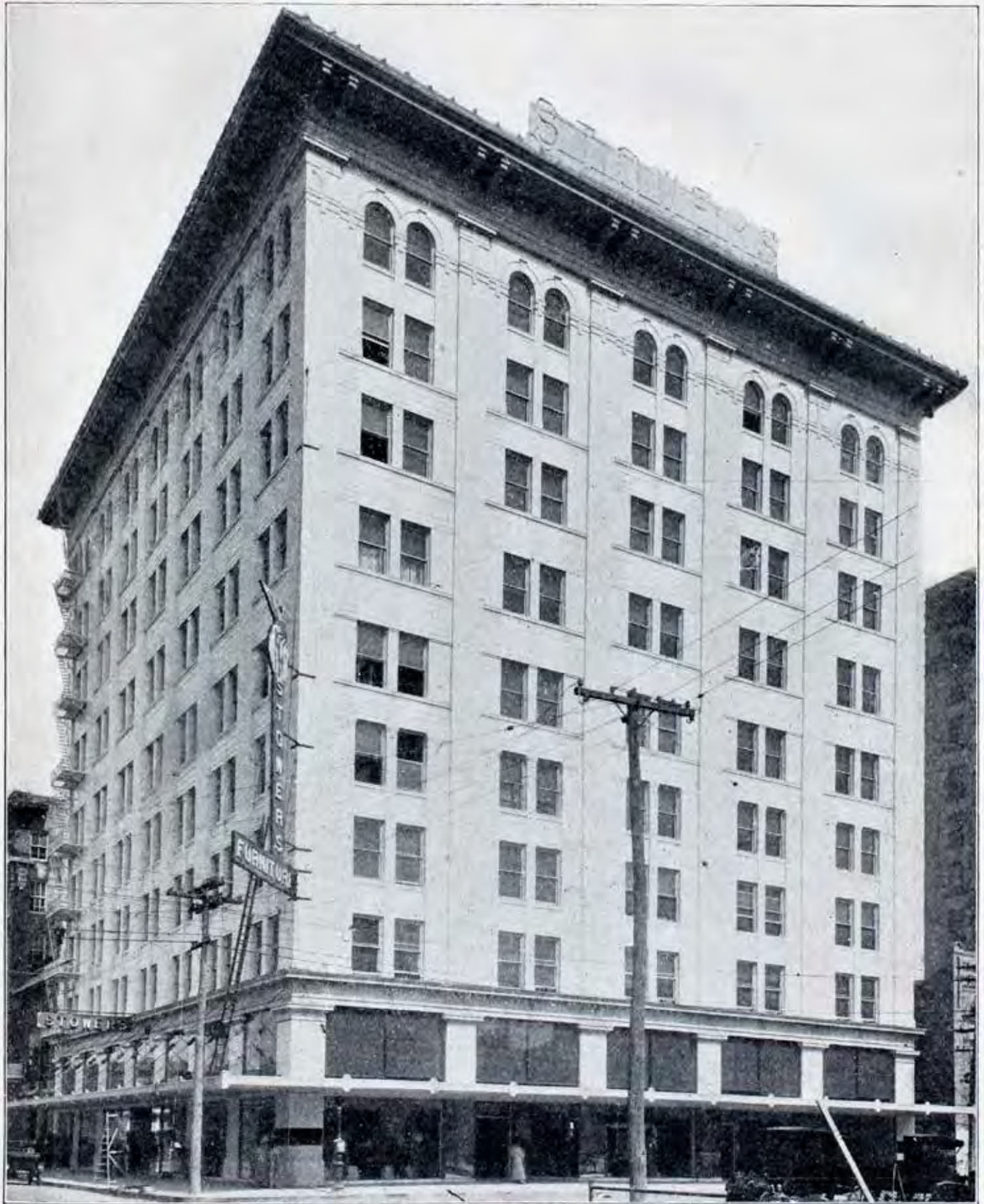
South (L) and east (R) elevations, view NW. Photo 1916 and courtesy: Illustrated Book of Houston , page 99. Houston Metropolitan Research Center, Houston Public Library (HMRC-HPL).
