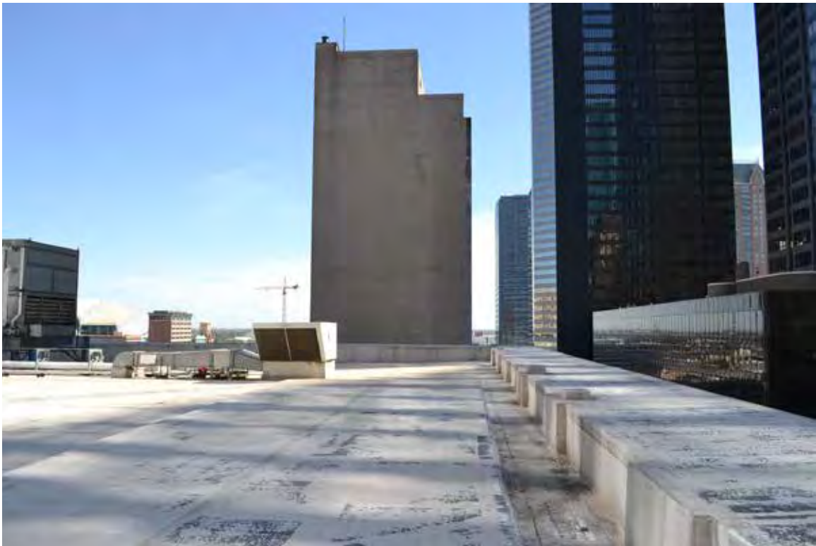
B: Roof, view E from SW corner. SWCA photo, 2014. File 0665
