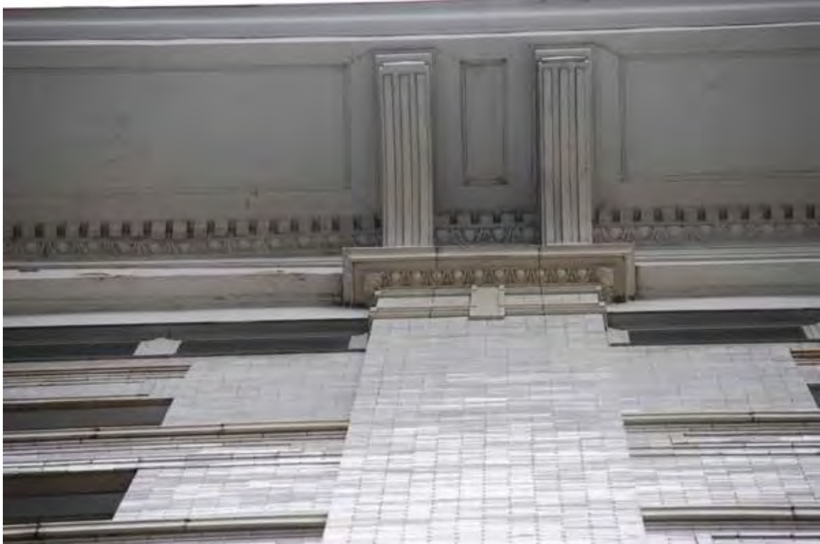
A: Detail of glazed brick, pilaster capital, and cornice. SWCA photo, 2014. File: 00_DSC_0159
