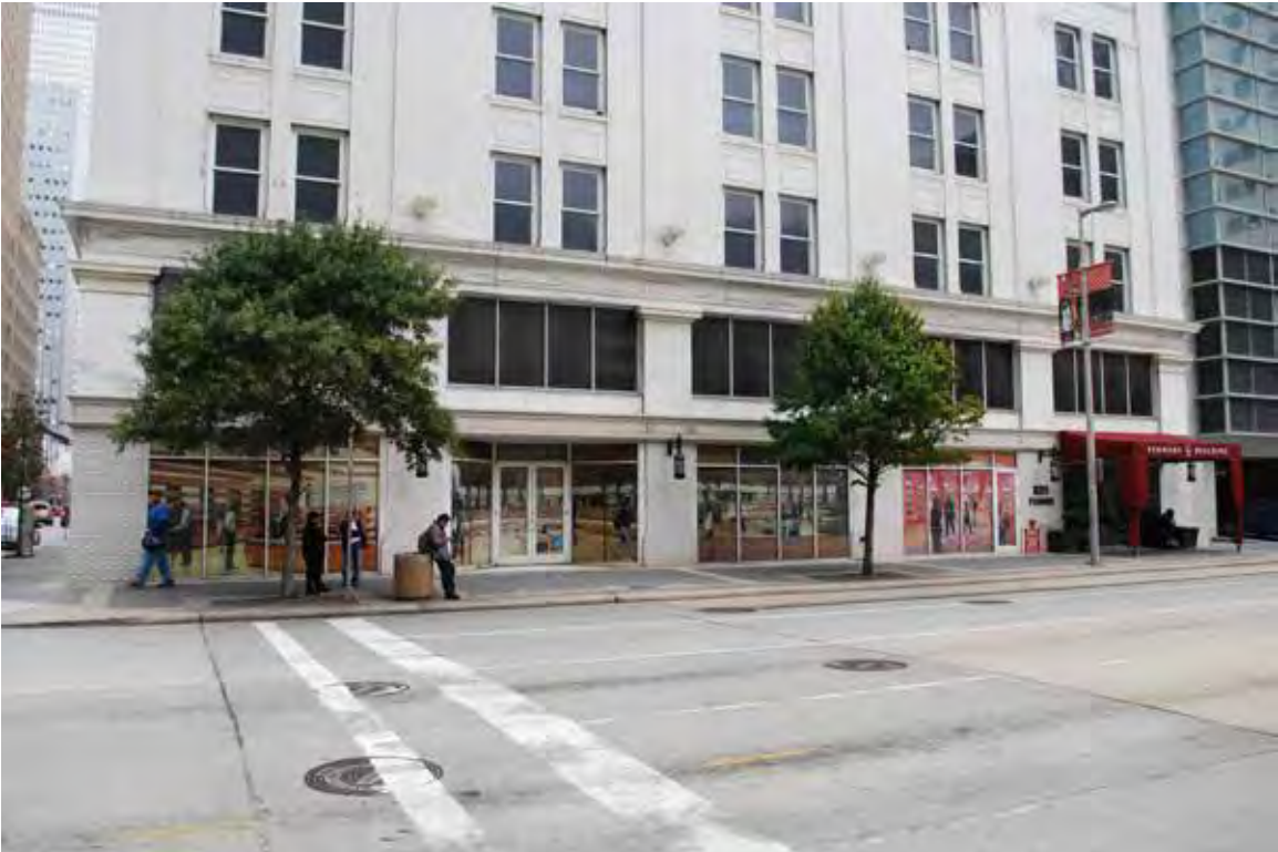
A: Detail E elevation storefront, view W. SWCA photo, 2014. File: 00_DSC_0178
