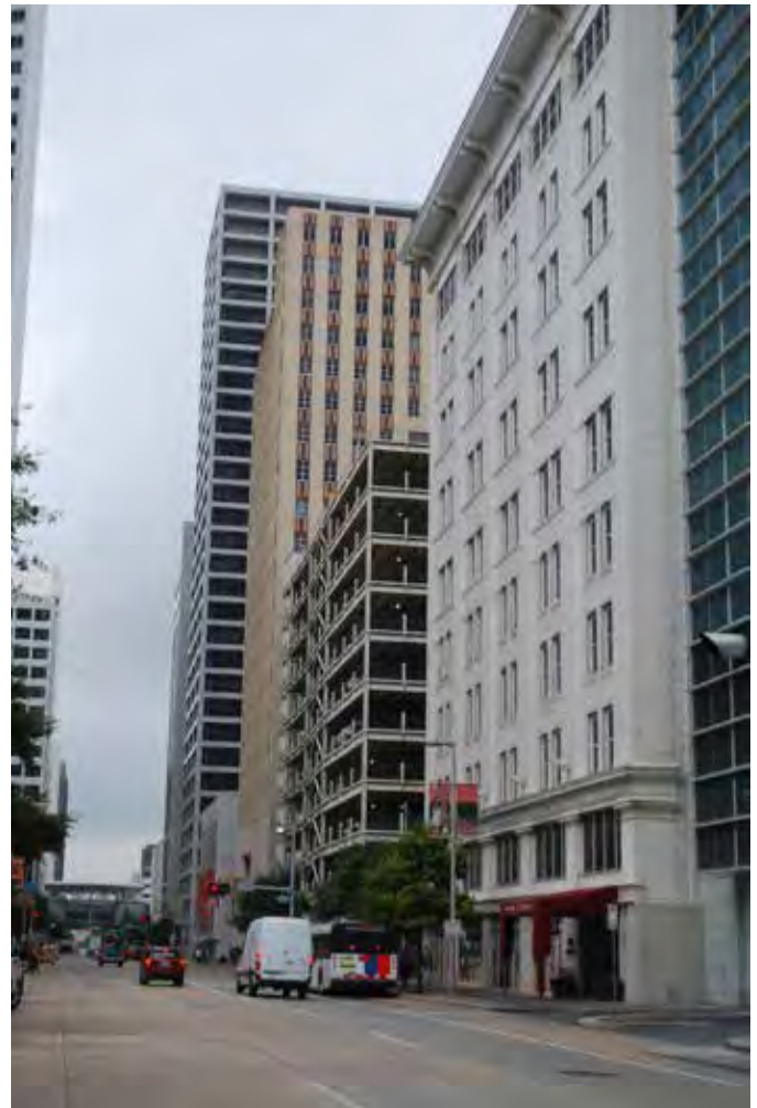
B: E elevation, view S down Fannin.
