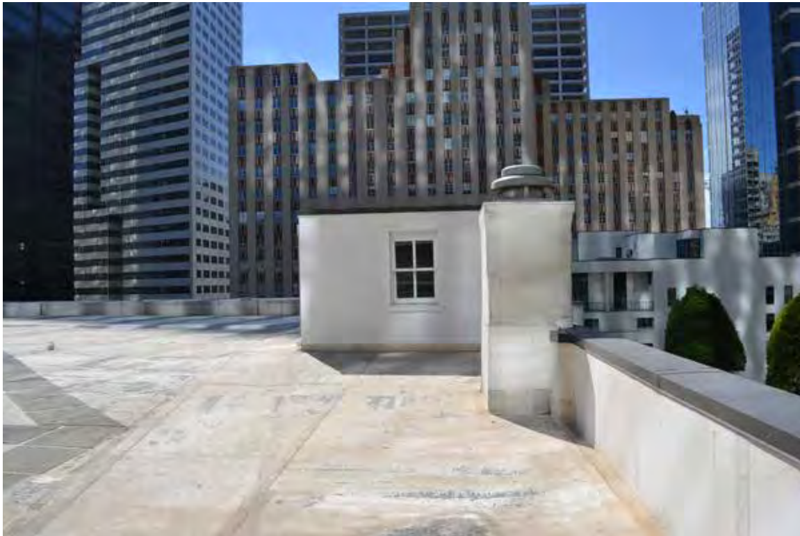
A: Roof, view S from NW corner. SWCA photo, 2014. File: 0663
