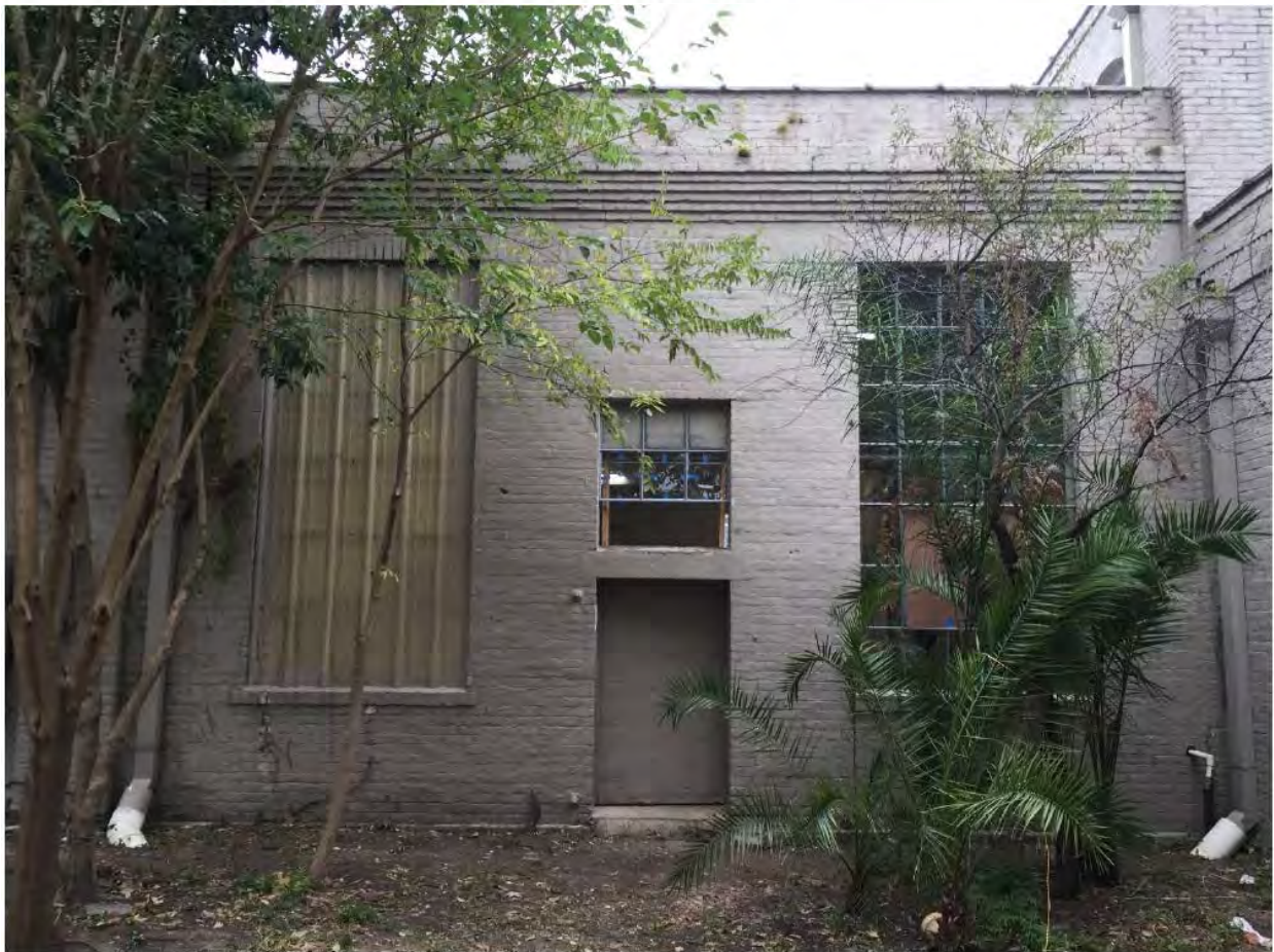
VIEW OF EXISTING HISTORIC METAL DOOR AND 6'-6" MASONRY OPENING. SOUTH ELEVATION
