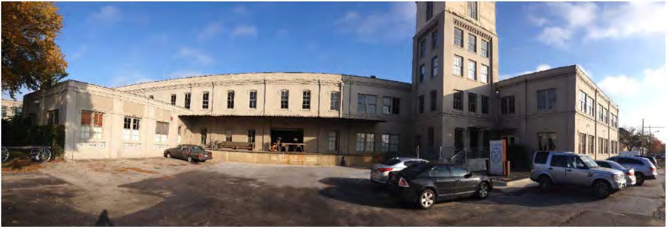
VIEW OF LOADING DOCK FROM W. 22 ND STREET, SOUTH ELEVATION
