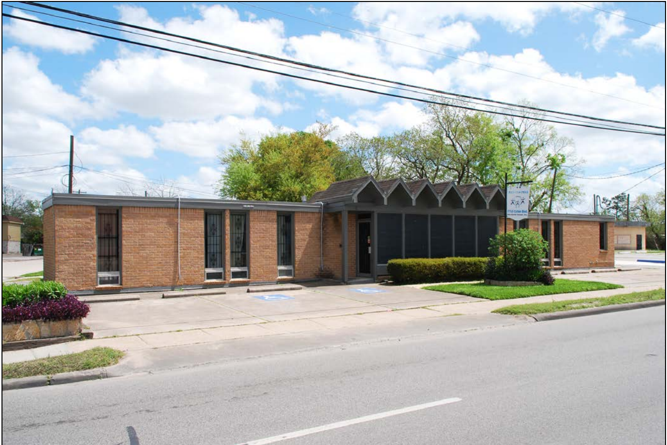
The Cullen Clinic, later known as Poindexter Dental, Inc., 7703 Cullen Blvd., Houston Architect: John S. Chase, AIA Year built: 1965 View: Front facade looking southeast
