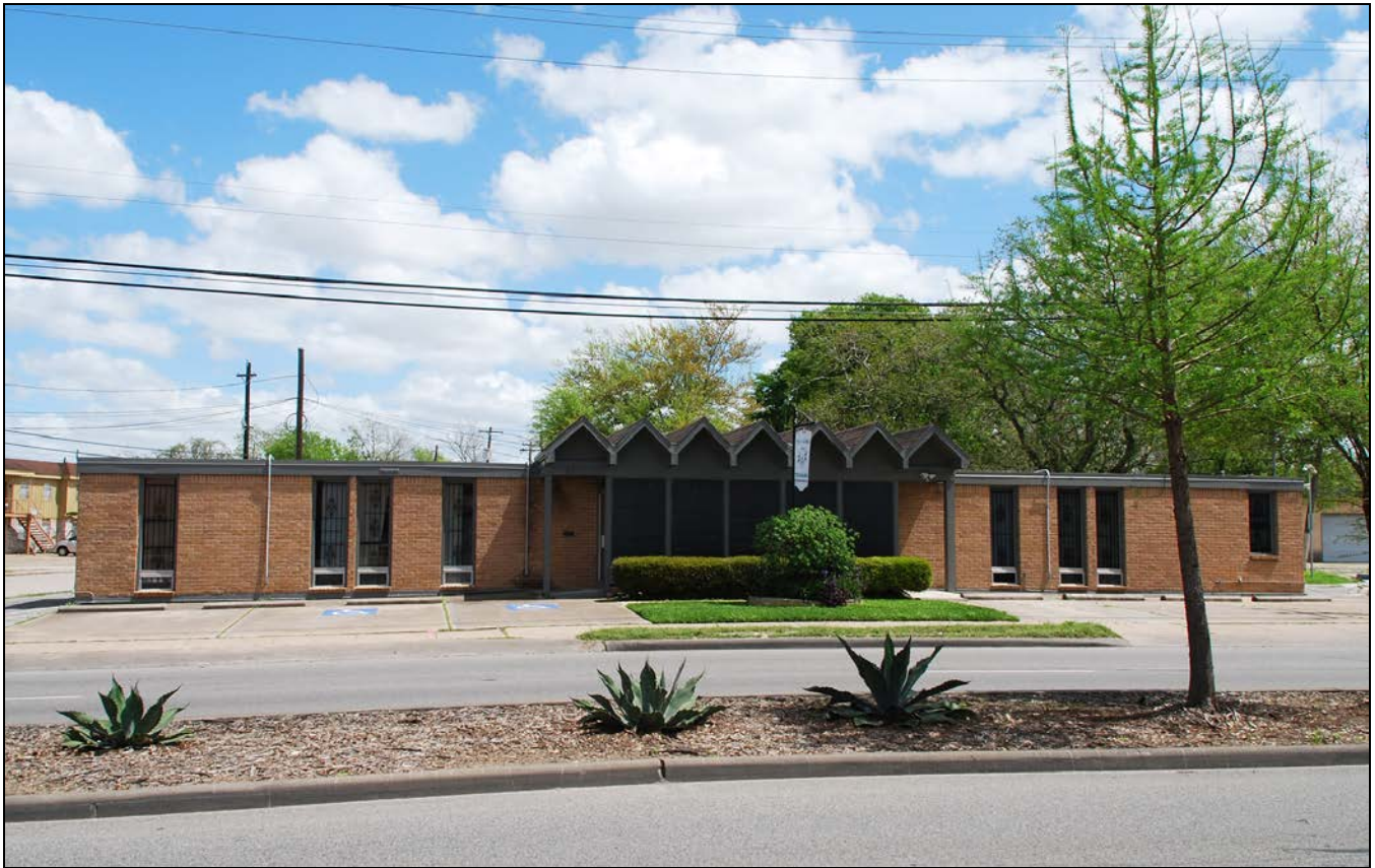
The Cullen Clinic, later known as Poindexter Dental, Inc. View: Looking east across Cullen Boulevard toward front facade Photos by David Bush, Preservation Houston Date: March 29, 2015
