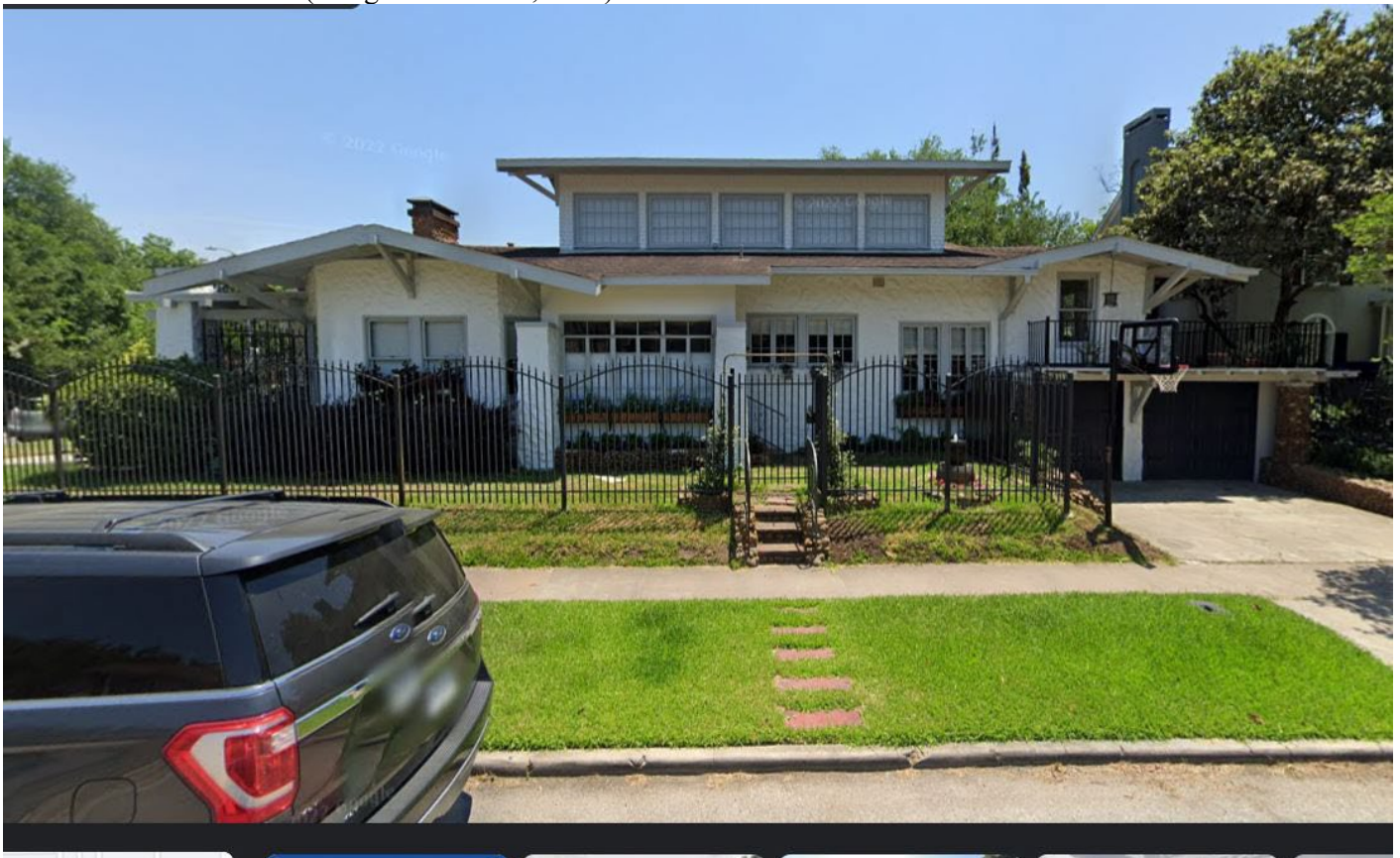
Photo 5: North elevation. (Google Streetview, 2023)
