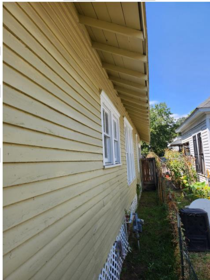
Left (North) Elevation Looking From Rear of the Lot
