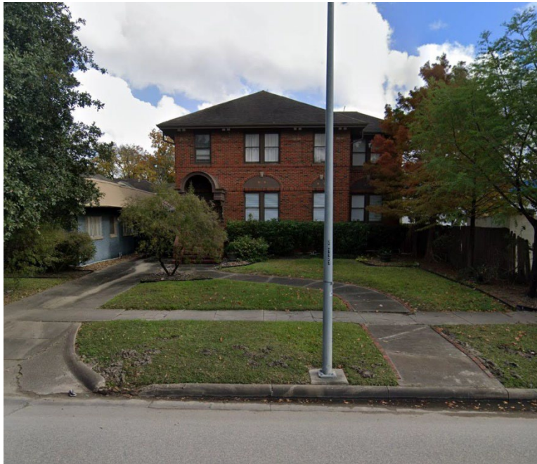
Non-contributing structure prior to demolition
