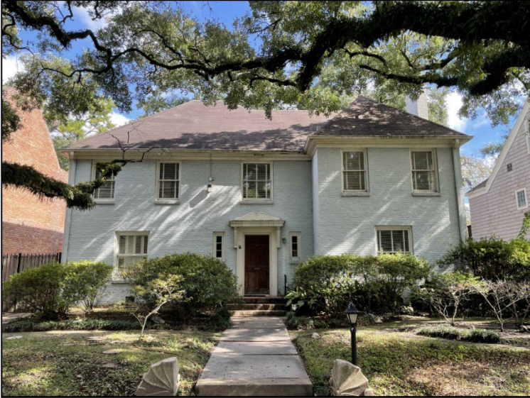
WEST ELEVATION AT MAIN HOUSE (FRONT FACADE FACING MANDELL)
