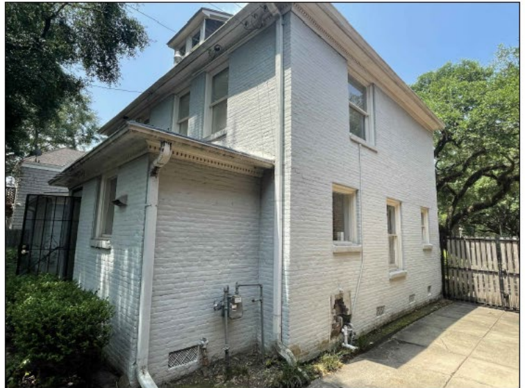
NORTH ELEVATION AT MAIN HOUSE (FROM DRIVEWAY)
