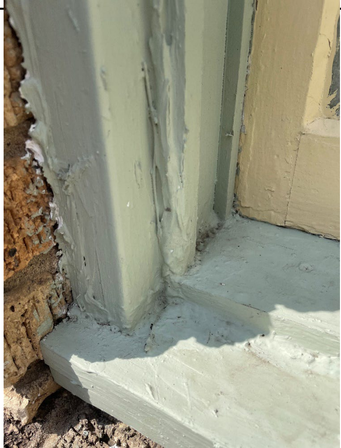
Figure 3 - Non-matching - non-orig. brick molding - damaged jambs, and sill
