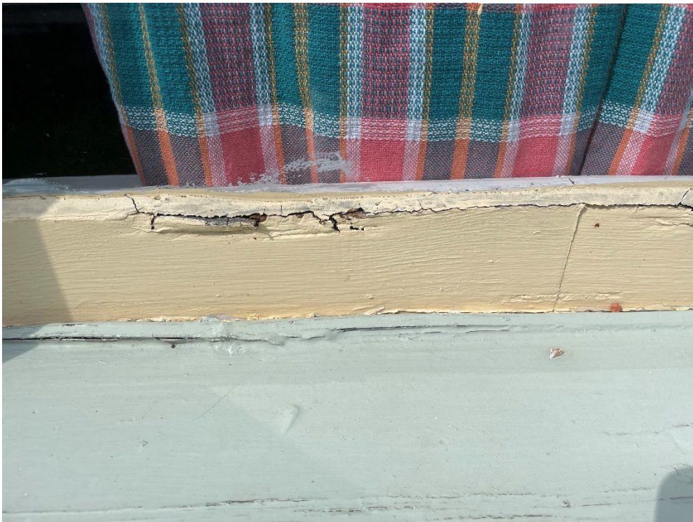
Figure 3 - Non-matching - non-orig. brick molding - damaged jambs, and sill
