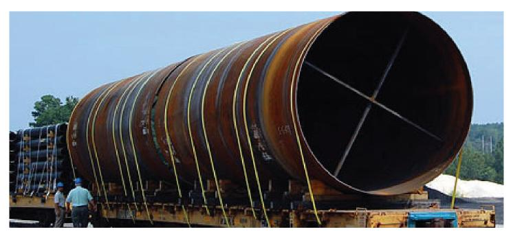
Two 108" pipes will carry the water from the intake pump station in Lake Houston to the Northeast Water Purification Plant facility.
