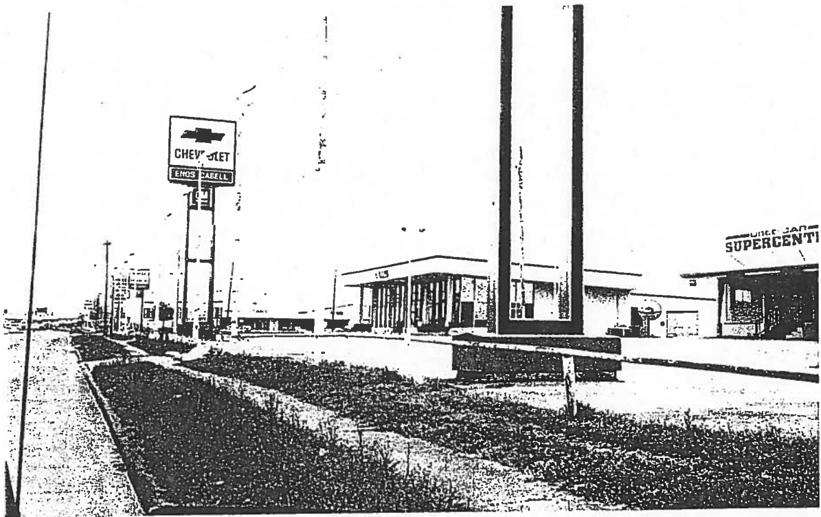
Figure 3B: 6800 Block Gulf Freeway – Vacant, boarded-up, deteriorating structures
