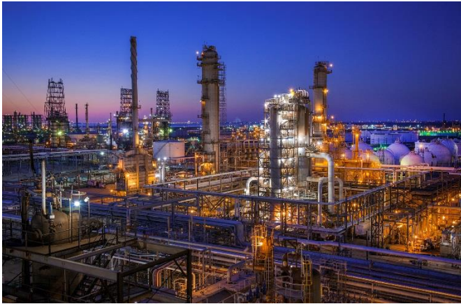
Petroleum refinery, Texas City, Galveston County
