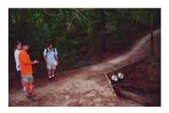
Trails should be aligned to avoid drainage ways, but where unavoidable, must be constructed to minimize impacts and maintain drainage flow without increasing erosion potential by sidetrailing. This solution in the Park channels bike traffic properly while minimizing the construction footprint.
