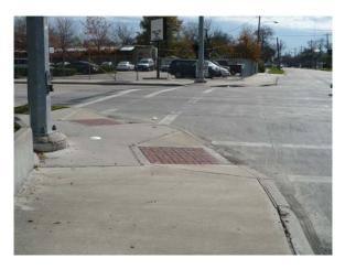
The intersection of Lyons Avenue and Gregg Street shows good sidewalk design. Although the striping is worn, crosswalks, ped signals and buttons, and ramps are provided in all directions. The sidewalks are wide and smooth.
