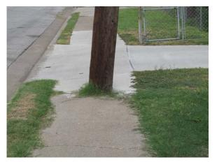
New driveway and sidewalk section leading into telephone pole.
