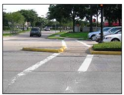
If traffic or signal timing requires pedestrians to cross the roadway one side at a time, median refuges provide a sense of safety. Cut-throughs can be at grade, or have a ramp at either end.
