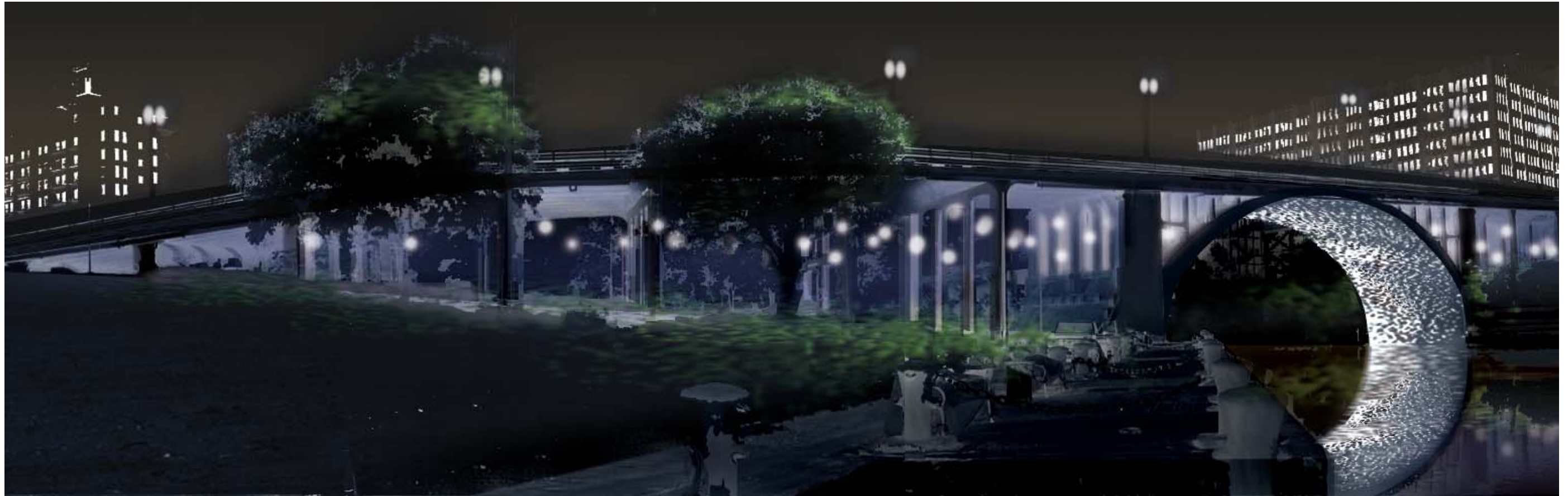
Main Street Bridge lighting treatments: reflections of water patterns cover the entire surface within the arch; white light within the arch structure radiates outward; point-sources among the bridge columns create an impression of glistening water. Photo panorama by Mary Edwards.
