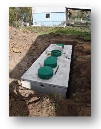
Figure 60 – OSSF being installed
