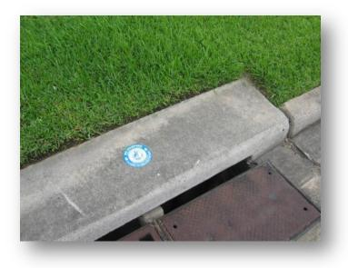
Figure 106 –Stormwater drain with marker
