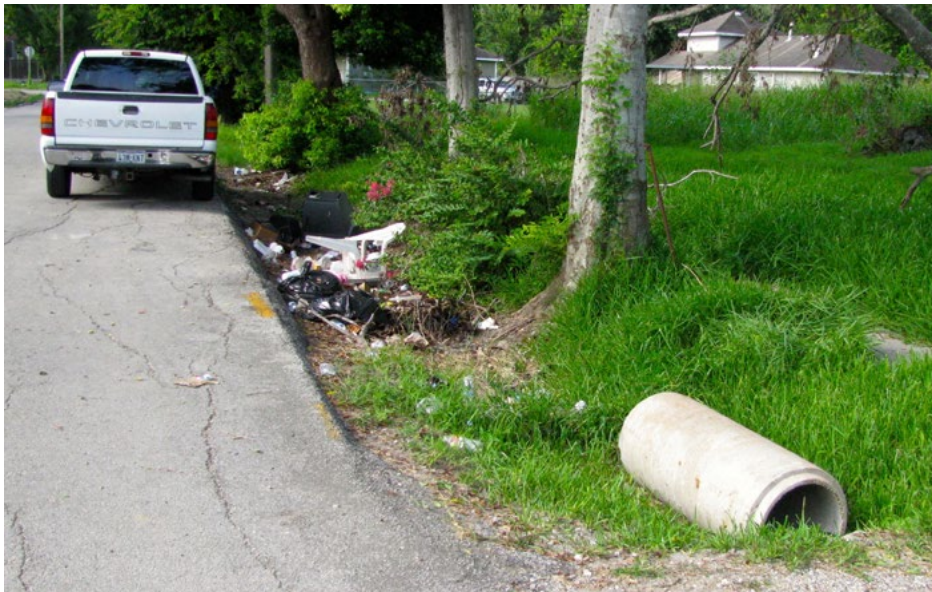
Overgrown and obstructed drainage ditch.
