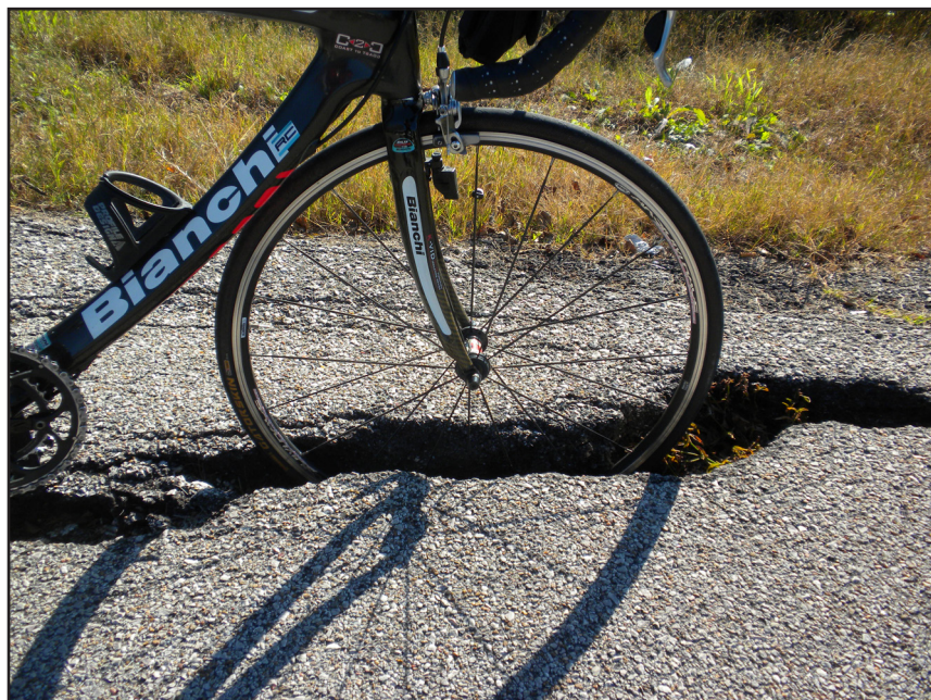
PHOTO 3: MEASUREMENT OF STREET CRACK DEPTH
