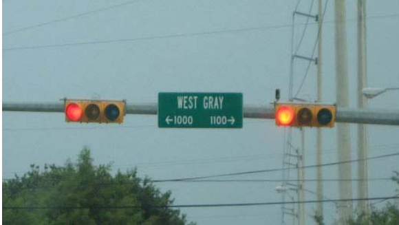
COH standard Street Signs mounted on signal arms where available to reduce clutter
