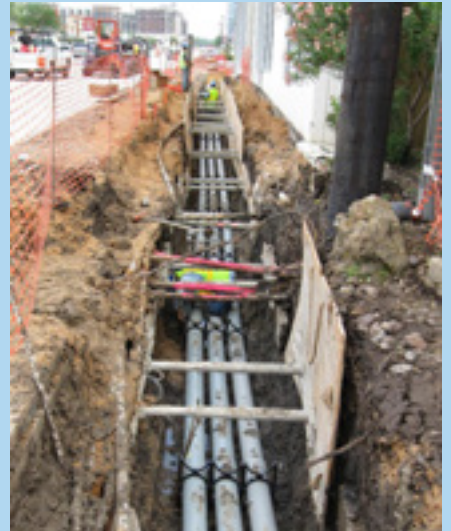
Underground utility ducts, construction phase
