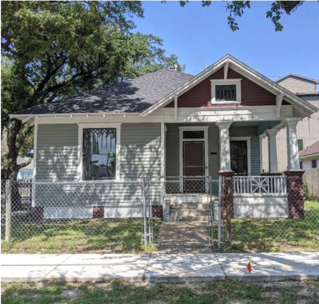
FRONT FAÇADE FACING CROCKETT STREET
