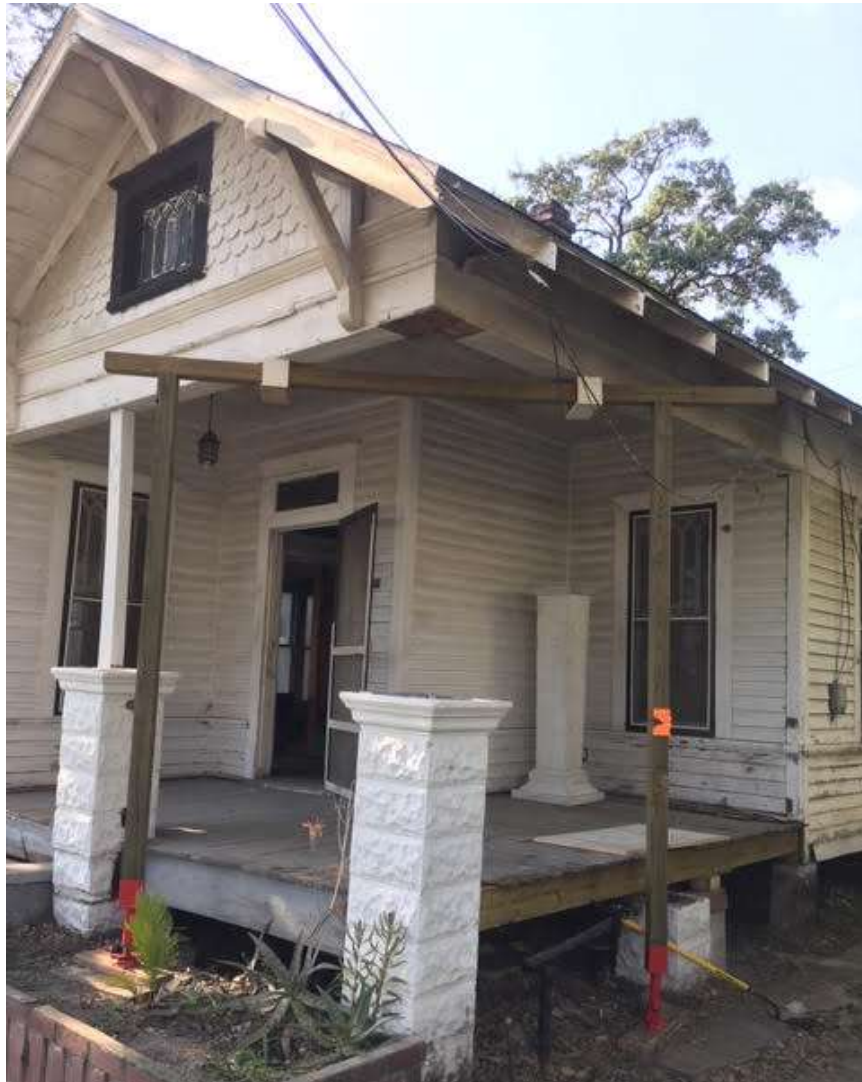
FRONT FAÇADE FACING CROCKETT STREET
