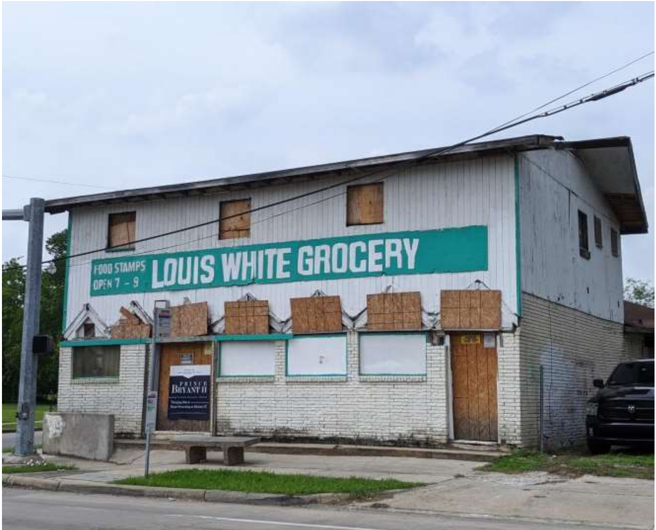
FAÇADE FACING LYONS AVENUE
