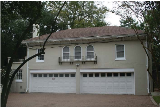
Carriage House – West Façade
