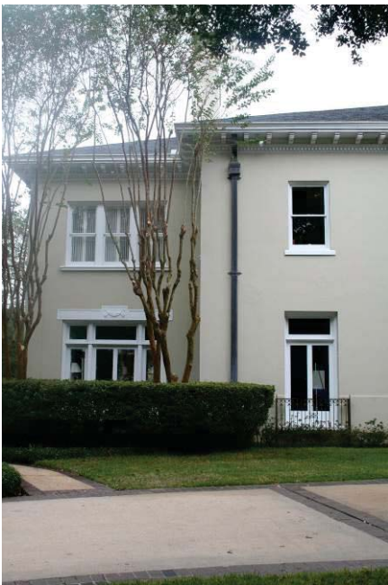
Front Façade – Northeast Corner
