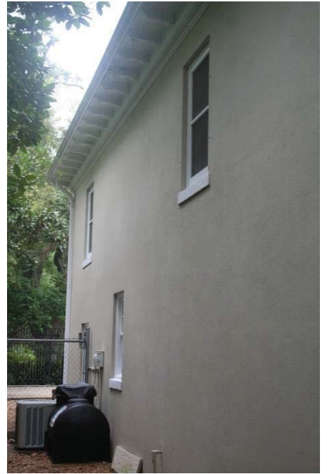
Carriage House – East Façade
