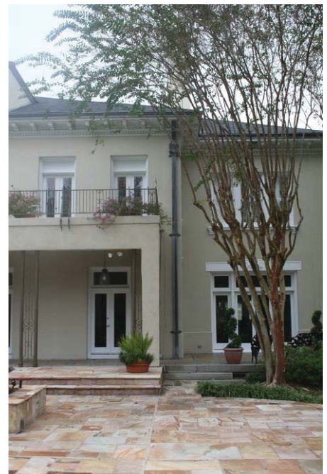
Rear Façade – Southeast Corner
