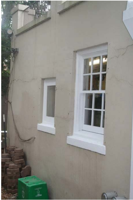
Carriage House – Southeast
