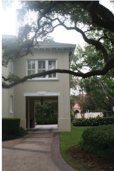
Front Façade – Northwest Corner
