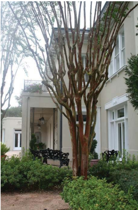
East Façade – South East Corner
