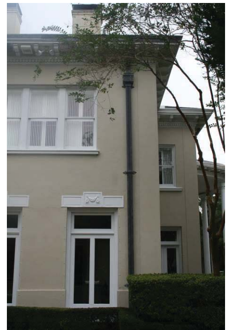
East Façade – Northeast Corner
