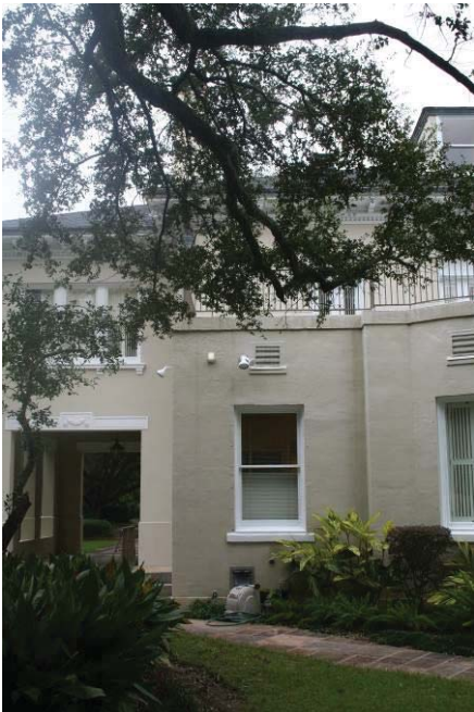
Rear Façade – Southwest Corner
