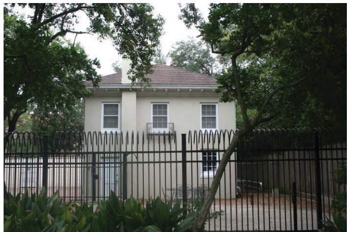
Carriage House – North Façade
