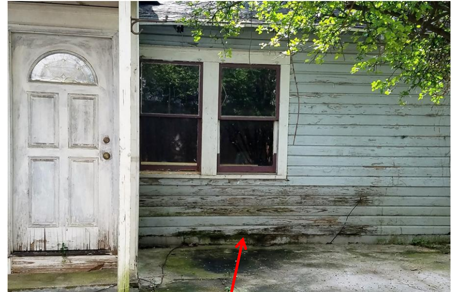
Flower shop (rear northeast corner of house) Propose to turn into an outdoor living / garden area; currently, significant water damage and rot
