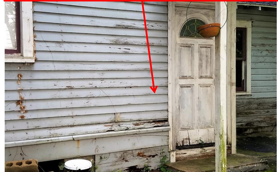
Flower shop (rear northeast corner of house) Propose to turn into an outdoor living / garden area; currently, significant water damage and rot
