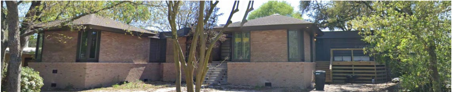
RENOVATION/ELEVATION WITH GARAGE ELEVATED C. 2020
