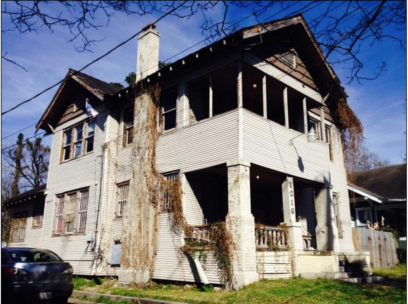
Condition prior to purchase and restoration.
