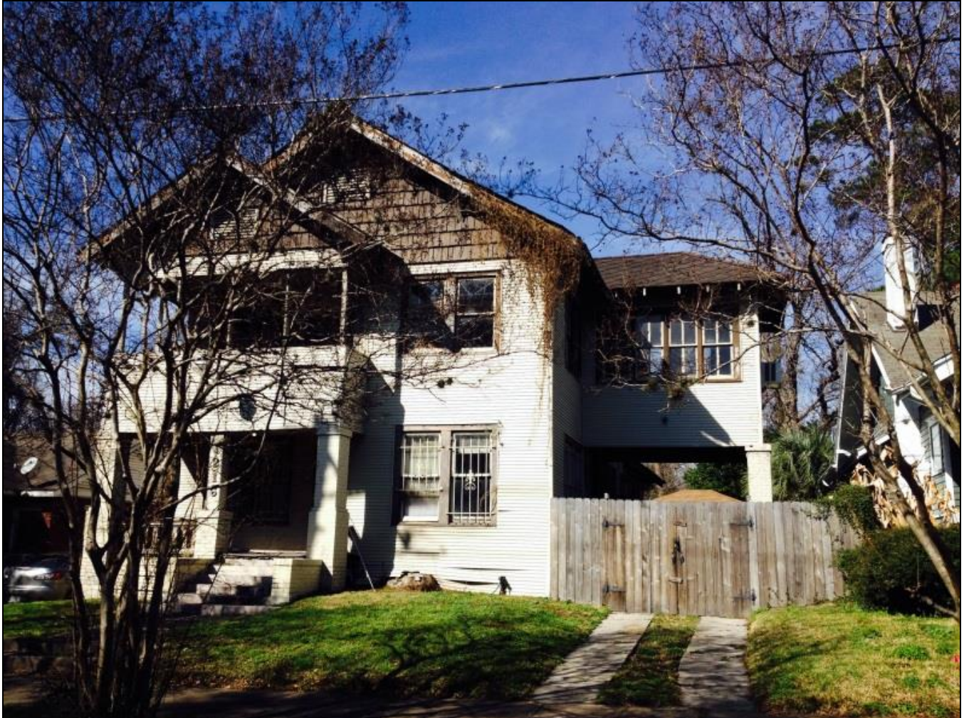
Condition prior to purchase and restoration.
