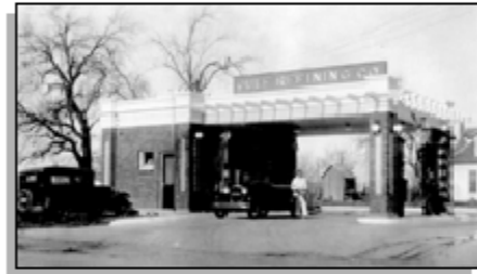
Figure 29: The above Gulf Refining Company station, located in Grapevine, is an example of the house with canopy form.
