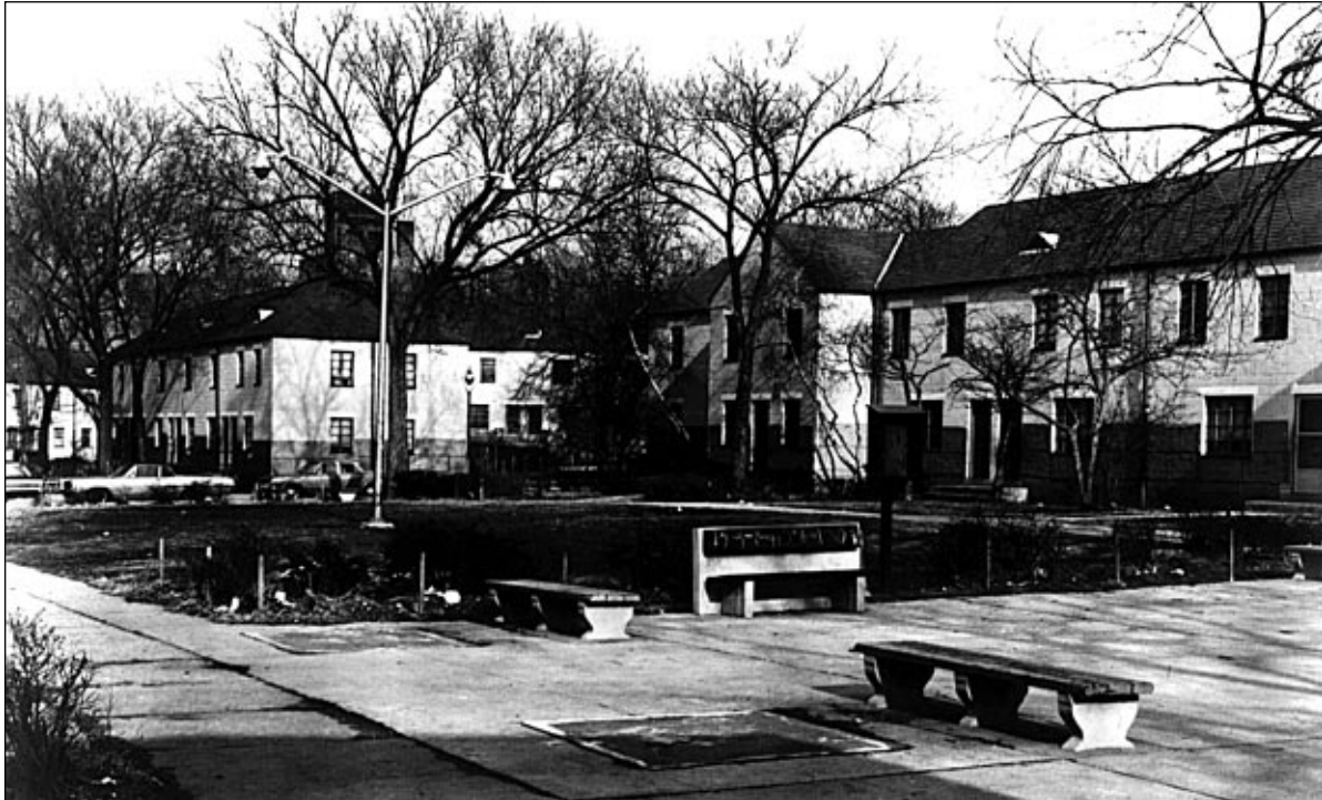
Figure III-9: The central area at Clason Point before modifications. This area was identified by residents and police as the most dangerous of the project.
