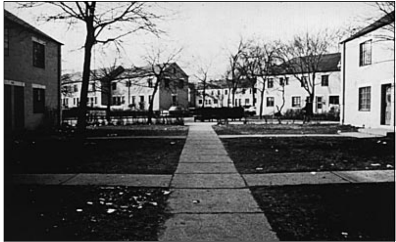
Figure III-2: Interior grounds of Clason Point before modifications.
