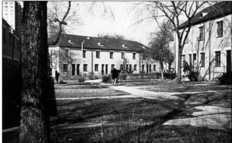
Figure III-13: View of internal walk at Clason Point before modifications.
