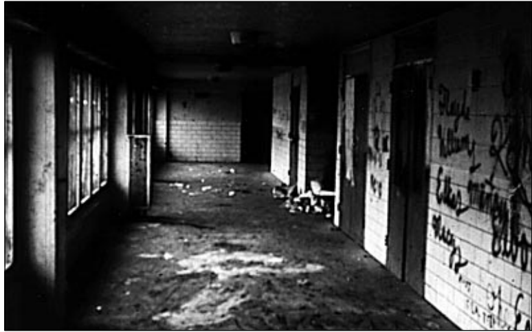
Figure I-3: The 3d floor communal corridor as it actually turned out, showing the vandalism that ensued.
