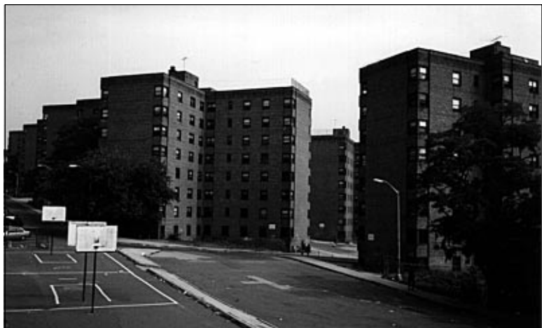
Figure IV-5: Existing public housing in Yonkers: the Schlobohm project.
