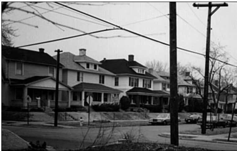
Figure II-2: Typical street in Five Oaks.
