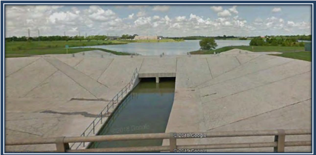
**Figure 35. Existing Outfall Structure at Brays Detention at Hwy 6**
