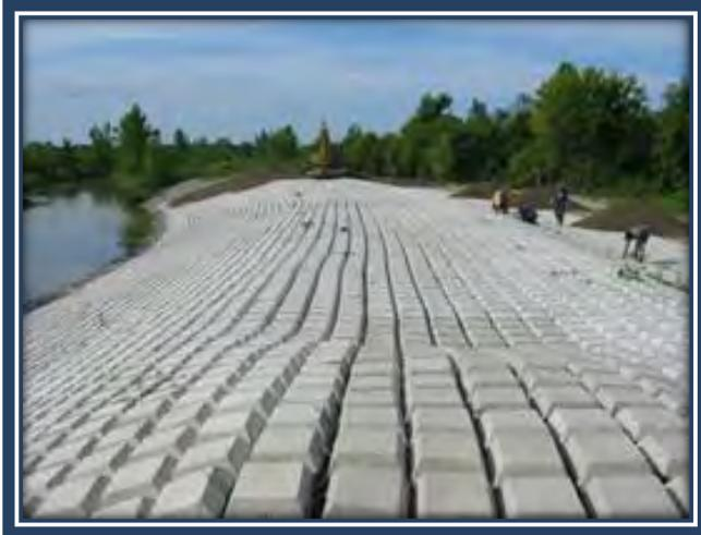
Figure 77. Articulate Concrete Block Mats ([www.environmental-expert.com](http://www.environmental-expert.com))
